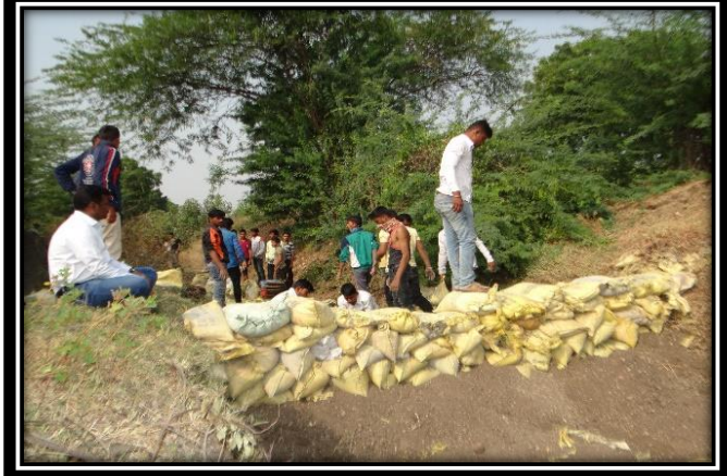
Gabion- Forest Embankment construction
