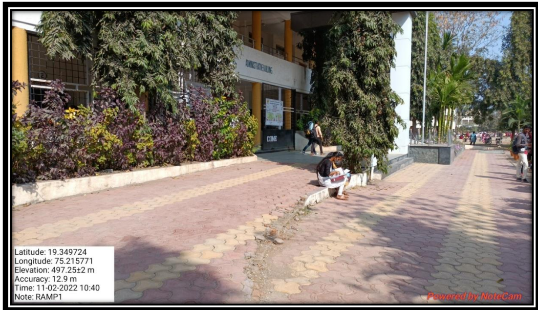
Ramp 1: Administrative Building
