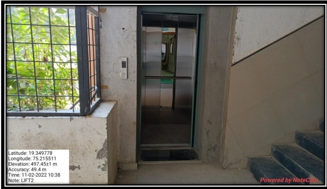
Lift: Internal View
